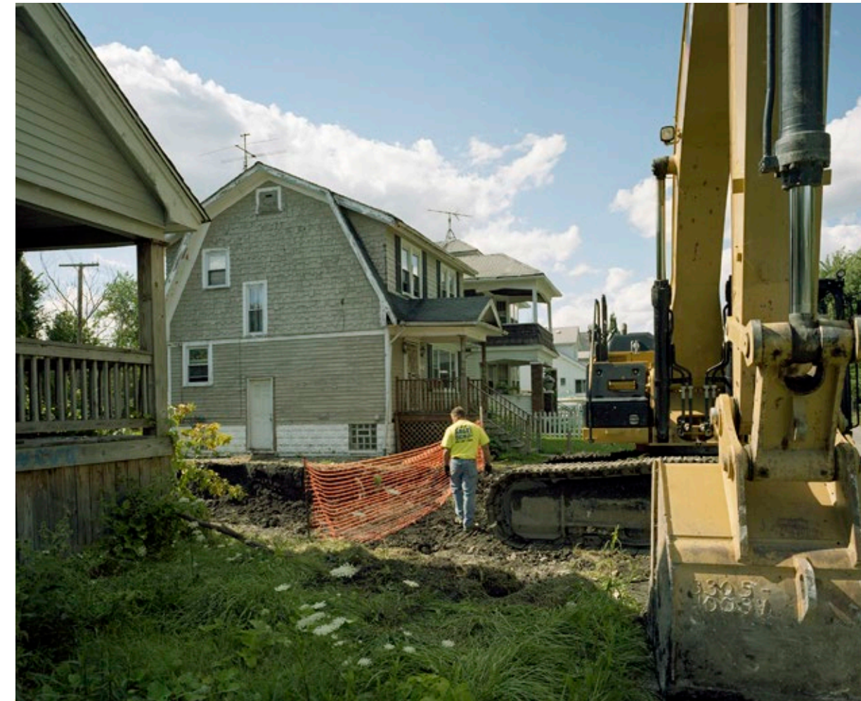
Legacy cities have unique opportunities house demolition and vacant land management with GI development. However, combining these processes can present governance challenges. PHOTO: CHRIS FAUST
