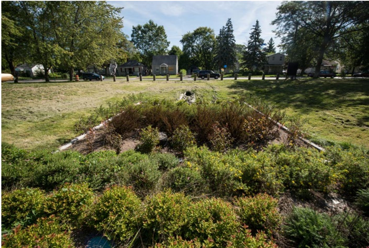
Residents often lack the tools, training or resources to conduct GI maintenance. This Detroit Water and Sewerage Department maintains this bioretention garden in a residential neighborhood. PHOTO: DAVE BRENNER
