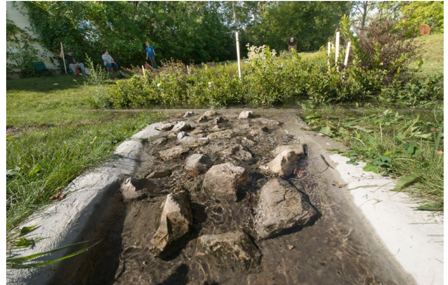
GI captures and manages stormwater using landscape features, rather than removing it only through a sewer system. PHOTO: DAVE BRENNER
